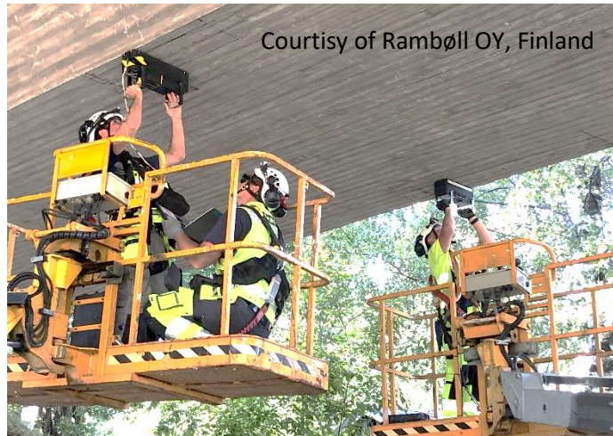
Implementaion of MIRA's for detection of voids in cable ducts, Finland
