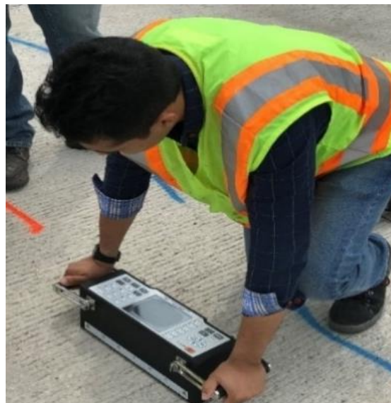
Implementaion of MIRA for detection bridge deck delamination, FHWA, Illinois, USA
