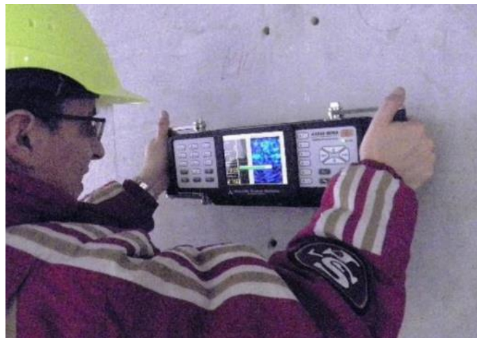
Implementaion of MIRA for detection of ungrouted element joints, Denmark
