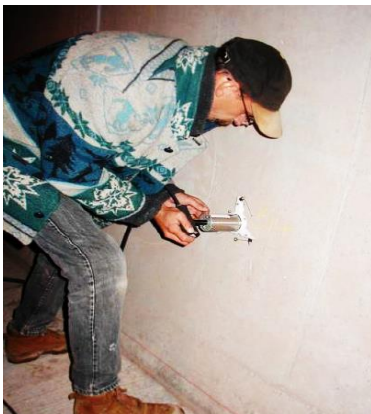
Tunnel thickness, Germany
