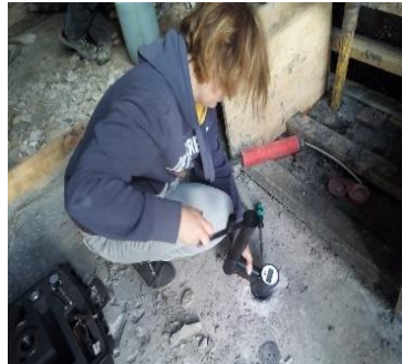
Tunnel Base, Denmark Strength before loading
