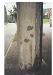
Highway bridge with deteriorating columns at the footings
