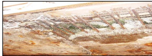
Severe cases of carbonation damage
