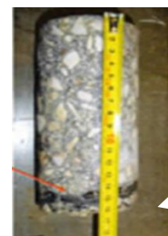
Filled out grout
