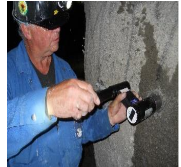
Shotcrete, Canada Strength
