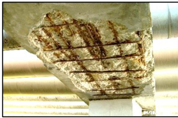
Severe cases of carbonation damage
