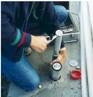
Industrial Floor, UK Strength before loading
