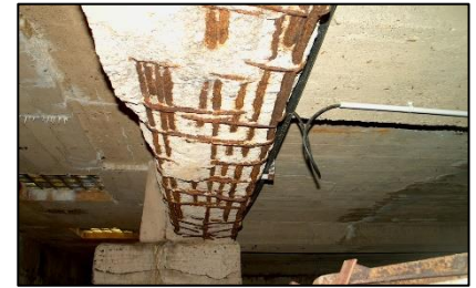
Severe cases of carbonation damage
