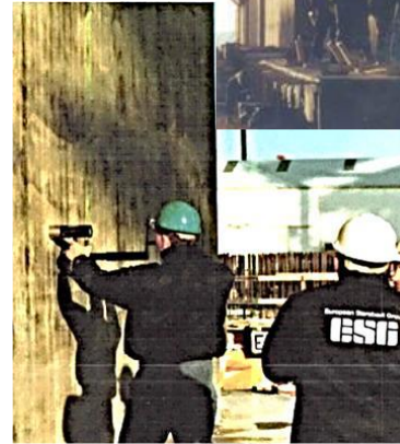
CAPO-test on the caissons of the West Bridge
