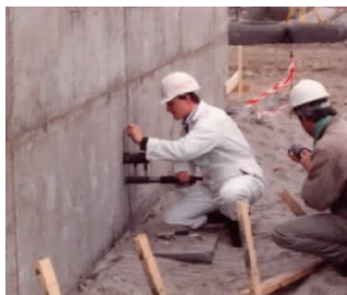
Supporting sea wall, Copenhagen Air cured. Pullout strength 70% of lab strength
