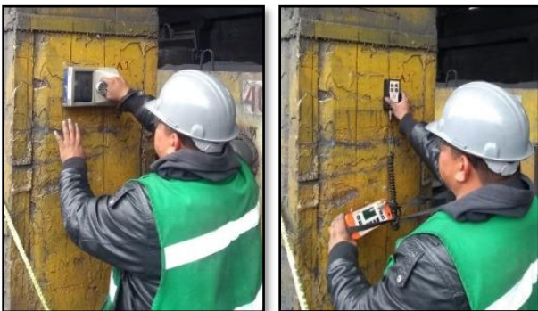
GPR for rebar depth Covermeter for size of bar
