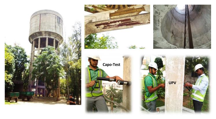
The water tanks that supply potable water to a part of city were built in late 1970s/ early 1980s. During this period, concrete was generally produced in small batches using portable mixers on the project location itself. The concrete was transported from the mixer and placed on site using manual labor.
