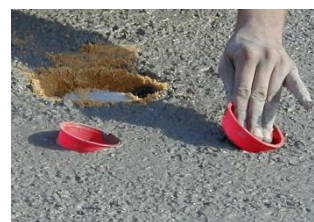
L-49 floating inserts being installed in the fresh concrete
