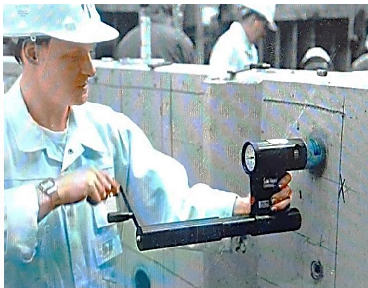
Certified CAPO-TEST technician Henrik Kristensen performing the CAPO-TEST on the tunnel elements.
