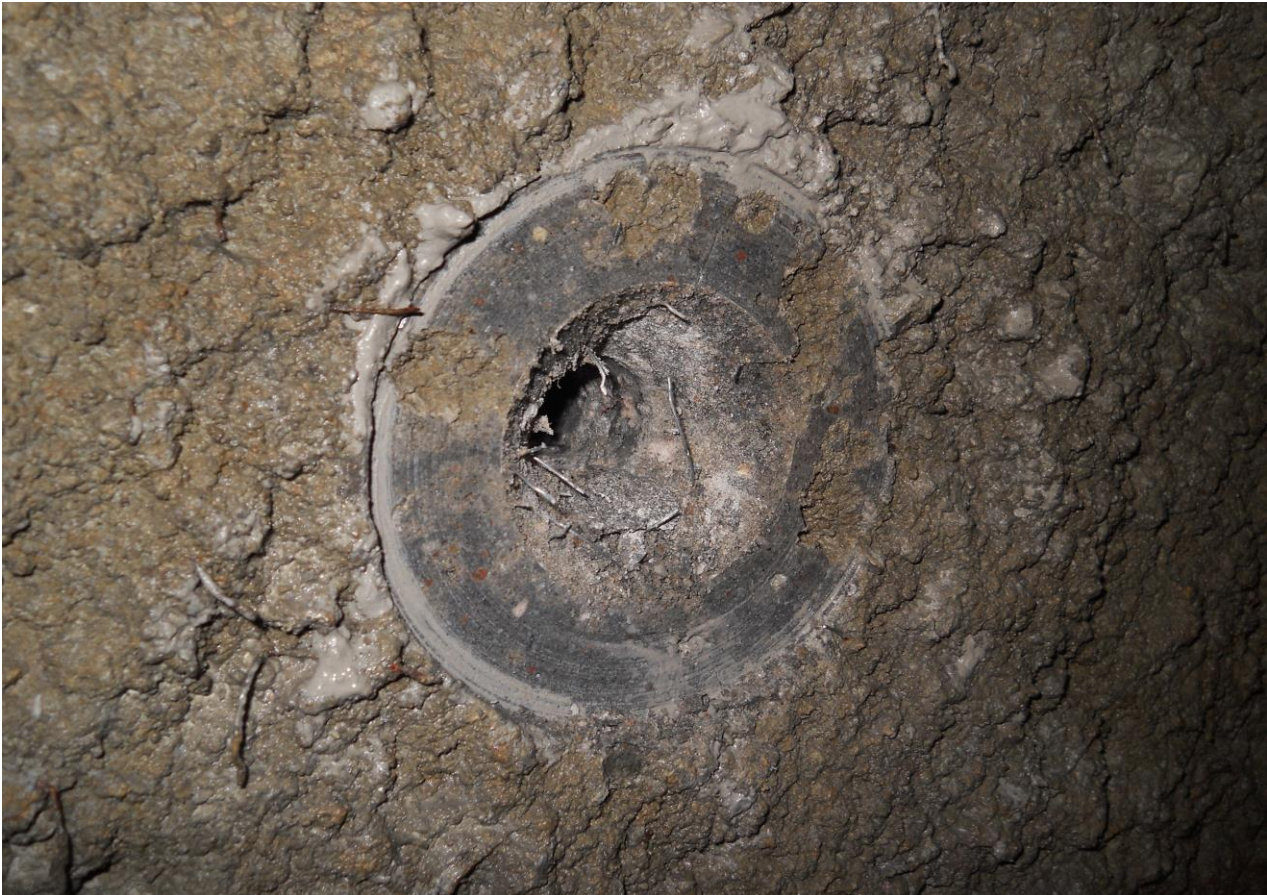
Capo-Test failure on shotcrete with steel fibers, fig. 12 Test results: 43.0 kN, 44.9 kN and 42.0 kN, shotcrete 5 weeks old
