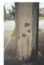
Highway bridge with deteriorating columns at the footings
