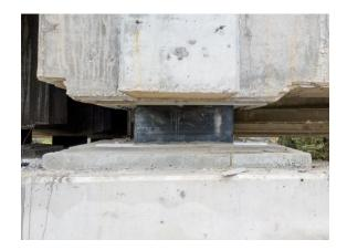
Finally, excessive deformations, bulging and oxidation of elastomeric bearings was performed with drones in a fast and efficient way with low cost.
