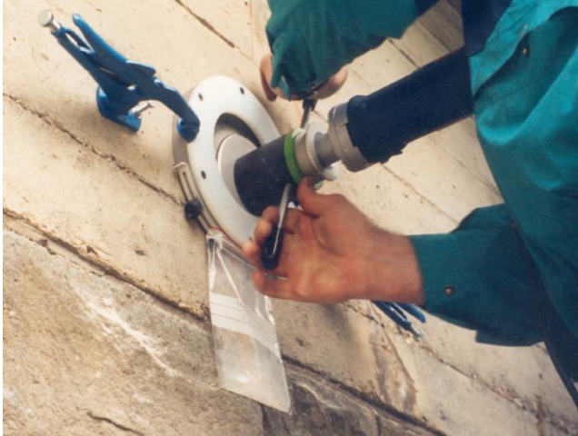
Profile grinding in progress
