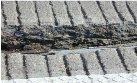
Example 1 of Freeze and Thaw cracking of the longitudinal joints of a concrete highway due to an improper air-void system in the presence of wet (saturated) concrete and freeze-thaw cycles.
