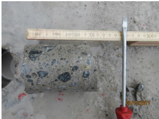
Core A. Intact 100 mm long with few fine cracks.
