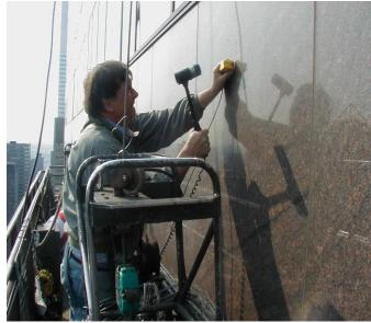
During construction of the high rise the granite panels had been fastened to a steel frame by means of 6 epoxy anchors. Holes had been drilled into the panels to half depth of the thickness, the anchors epoxied in the holes and subsequently fastened to the steel frame after which the frame sections were hoisted into position and fastened to the main steel structure.
