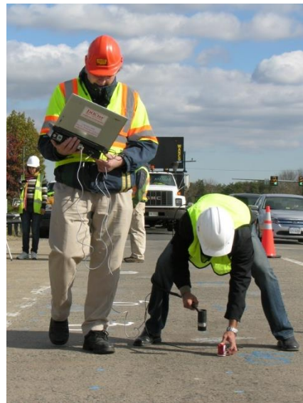
Testing for delaminations in bridge deck
