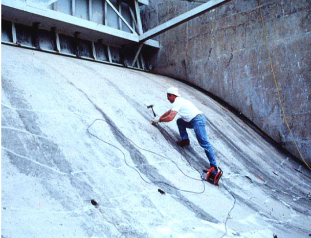
Testing for delaminations in dam spillway
