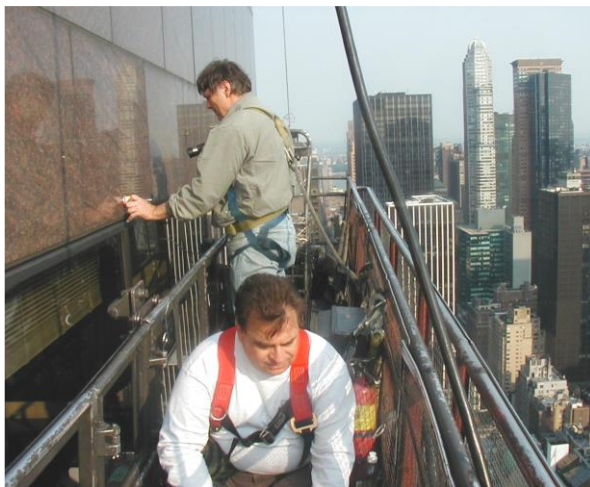
Testing for anchor integrity for granite panels in high-rise building
