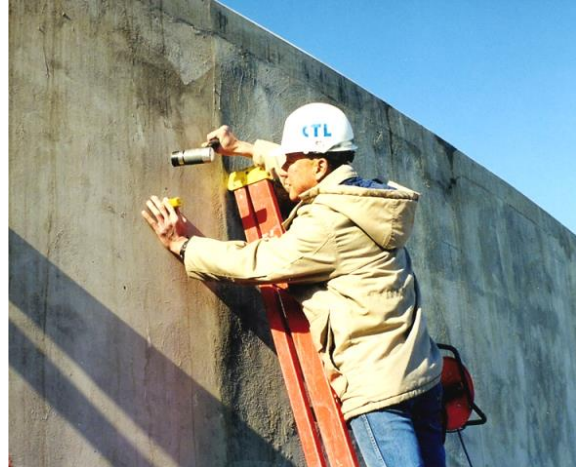
Testing for tightness of joints of concrete tank
