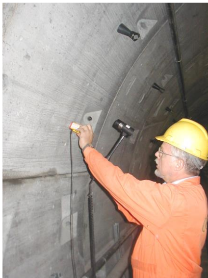
Testing for voids behind tunnel lining
