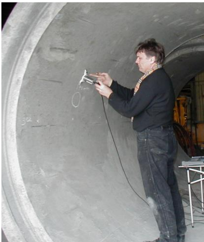
Detection of delaminations and honeycomb in sewer pipe
