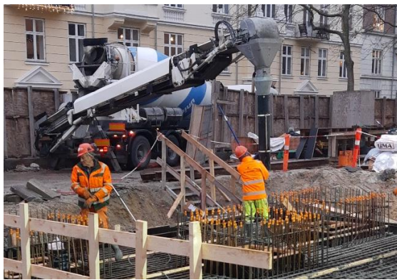
c) Cast concrete
