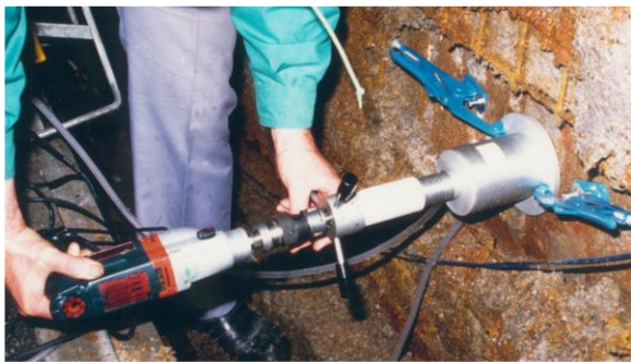
Coring with the CS-75 rig for inspection of cracks following chloride extraction
