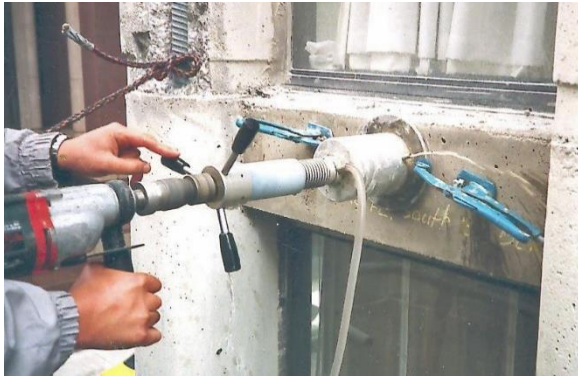
Coring with the CS-75 rig clamped to the surface
