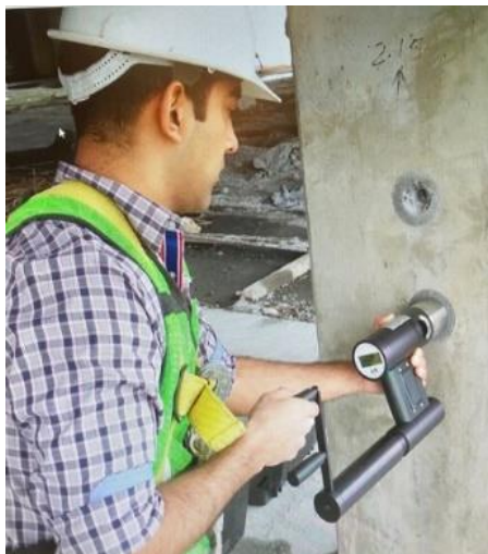
Column being tested for strength acceptance, Mexico
