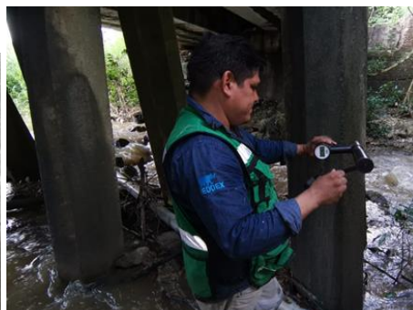
Structural evaluation of a railway bridge, Mexico
