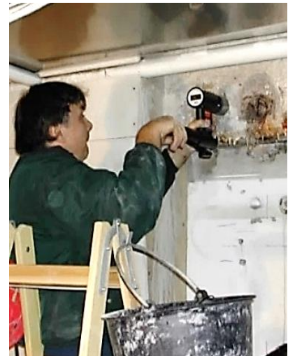
Dubious beam being tested for strength, Denmark
