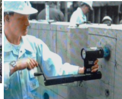
Quality assurance of tunnel lining segments, Channel Tunnel, UK
