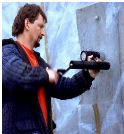
Testing the curing conditions of the "peel" protecting the reinforcement, Great Belt Link project, Denmark
