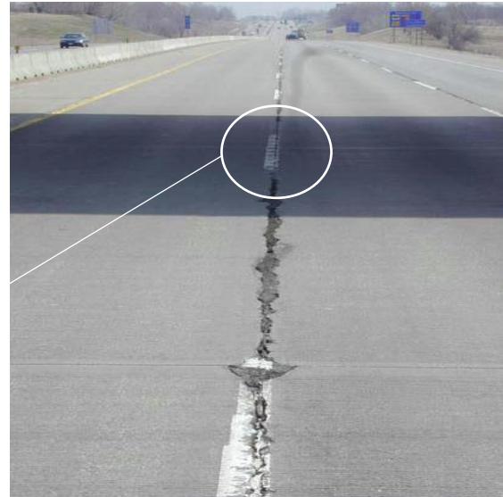
Centerline joint spalling of a highway after 10 years in service in a freeze-thaw environment due to improper air-void structure in the paste and presence of moist/water in the joints
